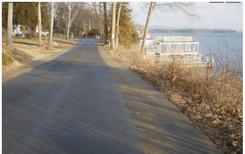
Assembly Point Road - little buffer, steep drop off on a road tilted towards the Lake
